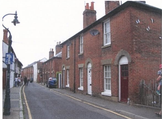
North side of Ivy Lane looking west
