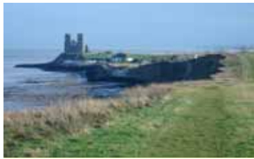
Eroding cliff line looking to Reculver Towers
