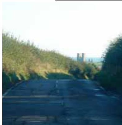
Creation of passing places on Reculver Lane
