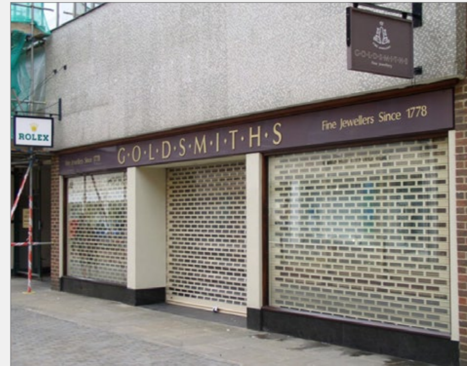
Image (left): Internal roller shutters on a former shopfront at 5 Rose Lane, Canterbury
