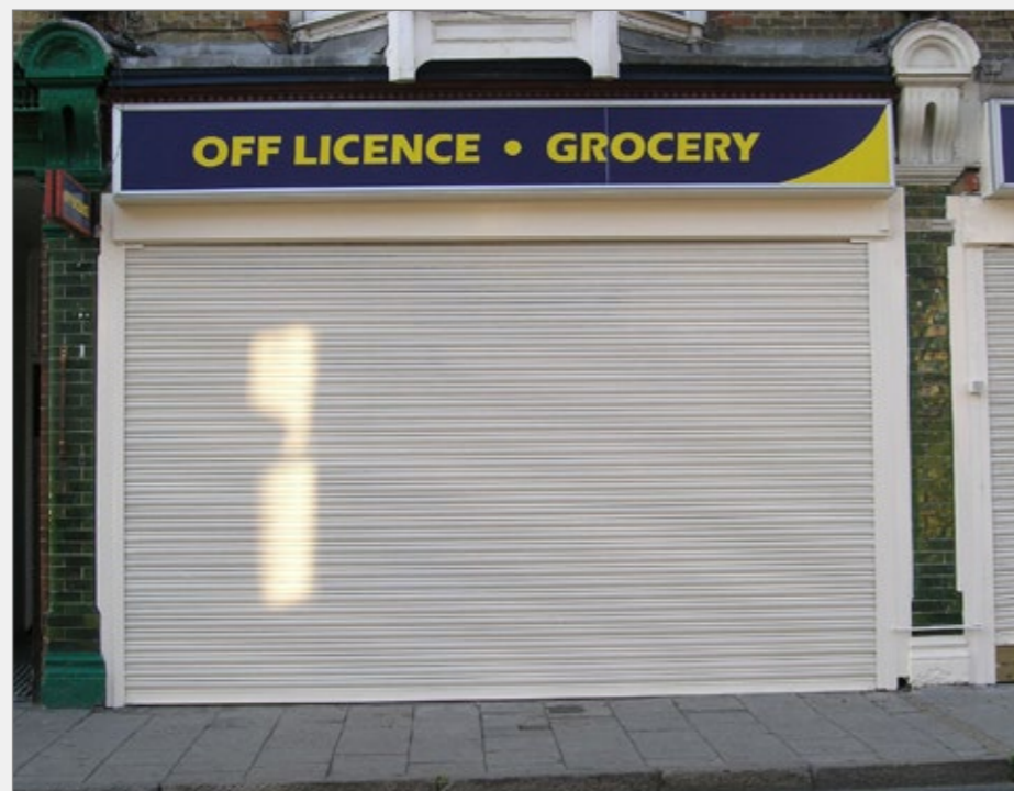
Image (right): Solid roller shutters obscuring the traditional shopfront: High Street, Herne Bay
