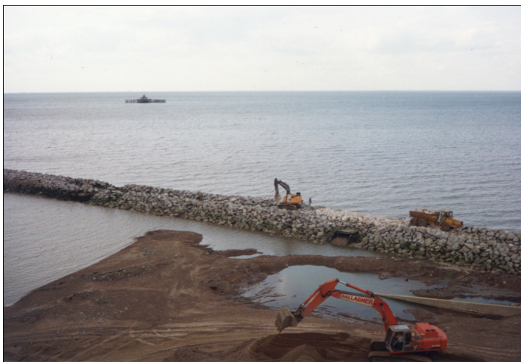
Figure 8.1 - Sea defences under construction at Herne Bay in 1990
