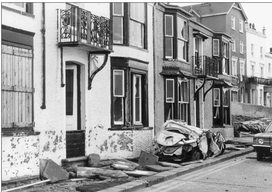
Figure 5.3 - Damage at Herne Bay as a result of the 1978 Storm
