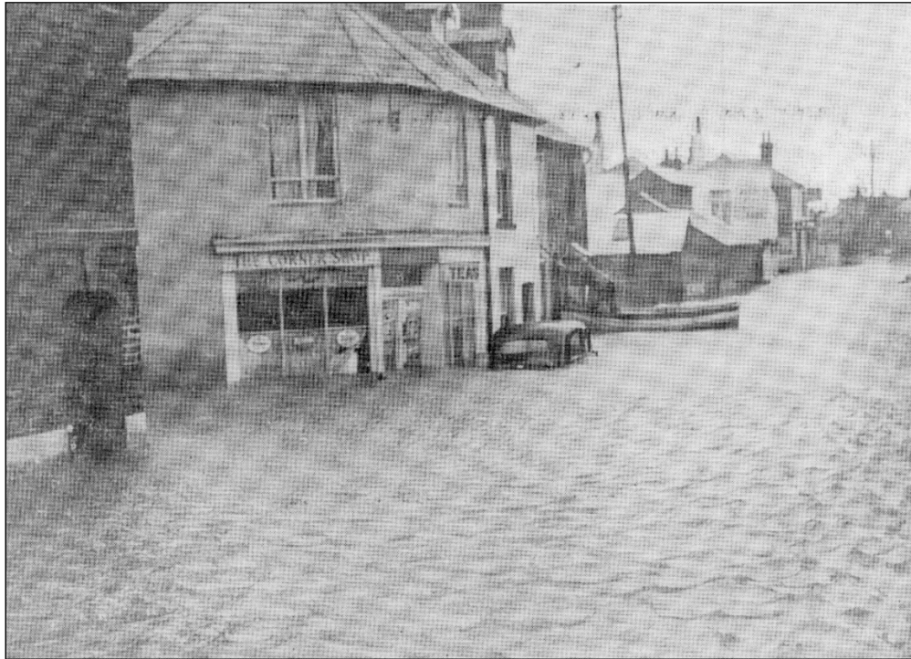
Figure 5.2 - Flooding at Whitstable, January 1953
