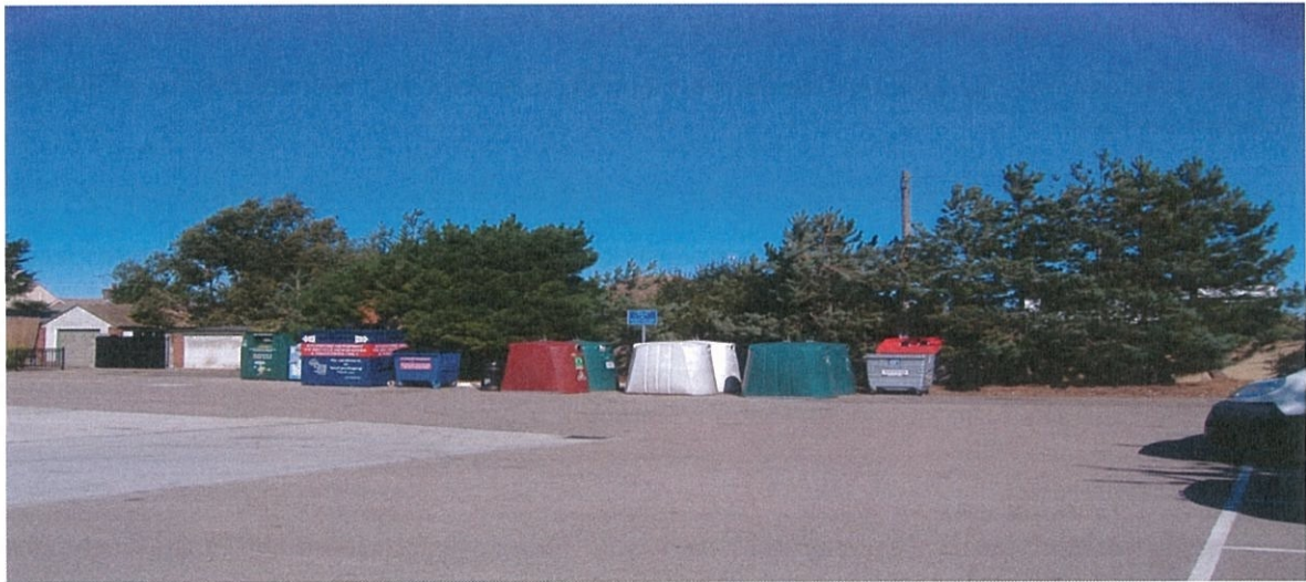
To the left are garages with access onto the '10 ft' right of way; recycling bins; trees; the substation is to the right
