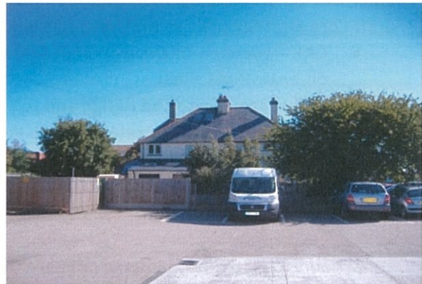
Rear elevation of 3 and 5 Pier Avenue
